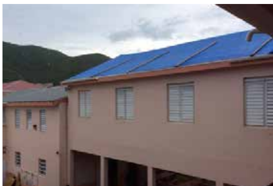
Roofs were damaged of two of the school buildings and repaired with plywood and tarpaulin.
